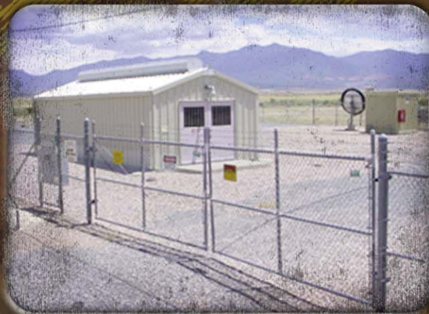
▲ METER STATION – FLOWING GAS
